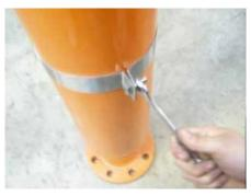
21. At the top of the stabilizer, tighten the bottom nut of the 90-degree elbow around the tubing using a 9/16" wrench.
