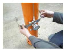
20. Secure the band by joining the ends together using the 3/8" bolt/nut and securing them with a 9/16" wrench.
